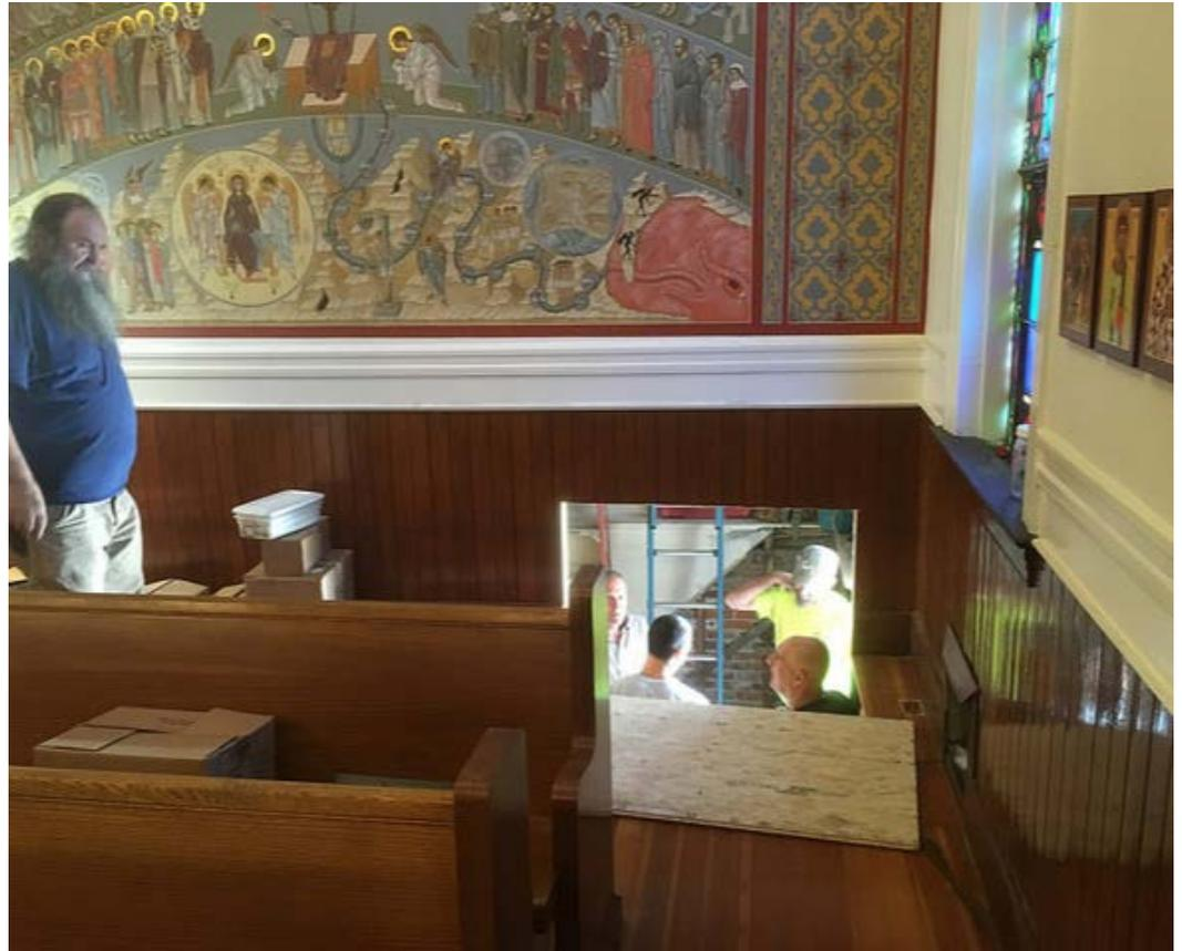
**Above: Cutting into the nave—very carefully!—for the bulkhead for the stairs.**
