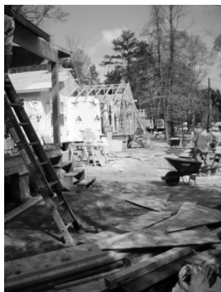
Pansy Street, St. Tammany West, the Habitat homes in progress.
