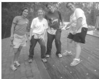
Half way done shingling--on the first side of the house!
