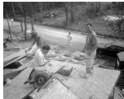
Despite the heat, they're still working hard on the roof.
