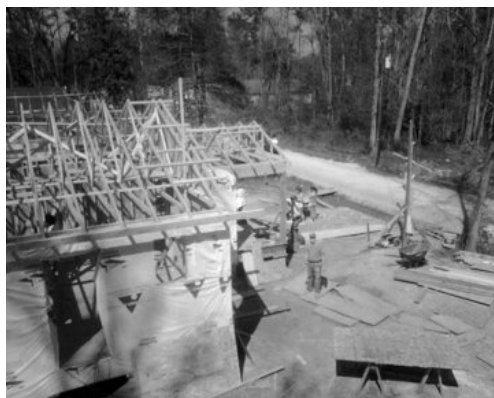
A rooftop view of the homes being built.
