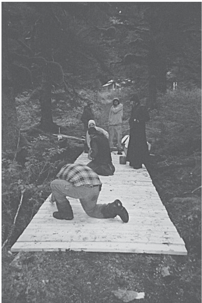
A new bridge being constructed
